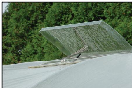
**Figure 18.** This rooftop vent allows hot air to escape when additional ventilation is needed on extremely hot and humid days.
