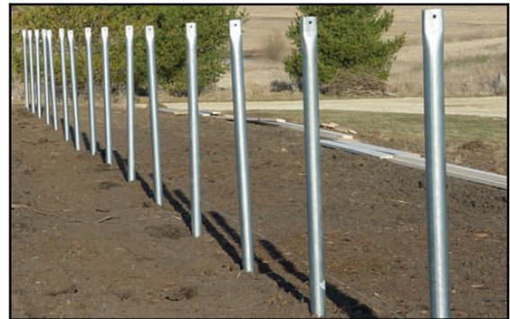
**Figure 1.** In Iowa, space posts every four feet, as opposed to the recommended six feet.
