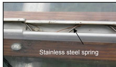
**Figure 10.** Stainless steel springs, tucked in an aluminum channel on the hip boards, offer continuous force along the surface of the plastic, are relatively easy to install and do not tear the plastic.
