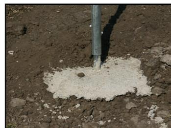
**Figure 2.** Post set in concrete.
