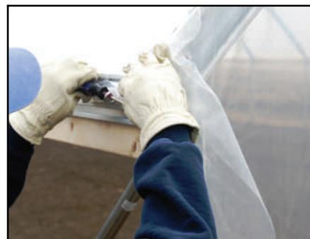
**Figure 9.** Fasten the plastic to the side or hip boards, mounted approximately 5 feet above the soil line on each side of the tunnel.
