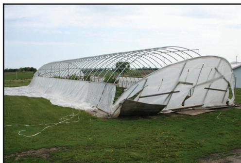
**Figure 3.** A windbreak can prevent serious damage caused by strong winds.
