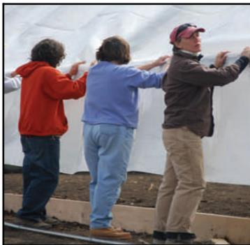
**Figure 8.** Several people located along each side make it easier to unfold and secure the plastic.
