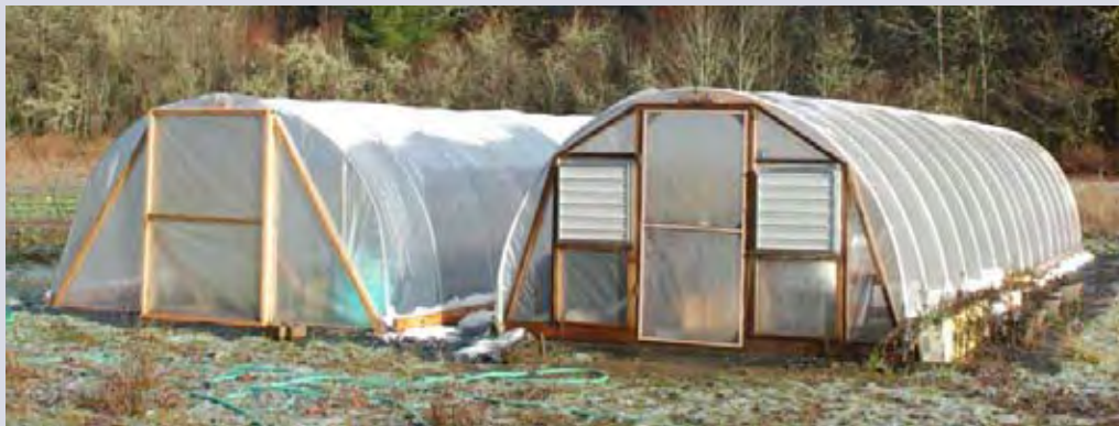
A PVC framed hoophouse and a cheaper conduit pipe design (left), both have been withstanding heavy winds and rain. Photo by Nick Andrews
